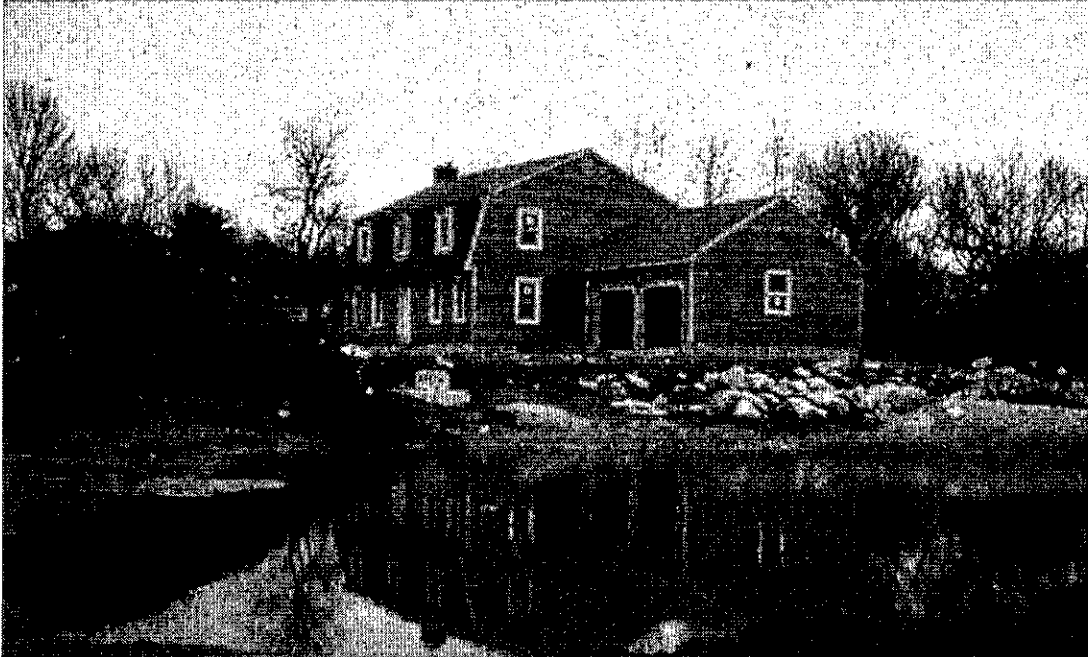
Figure 9. Septic system drainage fields will fail and basements may be wet on soils with mottled or gray subsoil and slow permeability.
